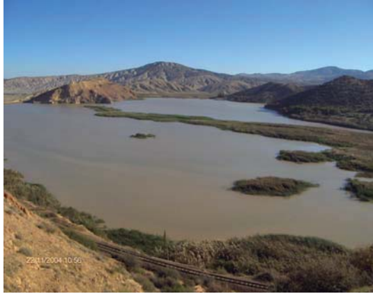
Fig. 2 Example of silted dam (Fergoug: we see that the basin is silted)
