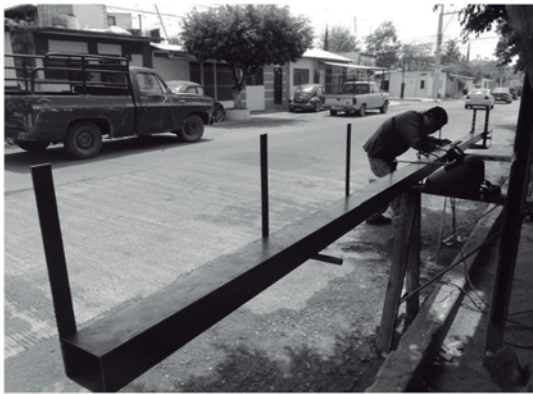
Fig. 1 Metallic PTR for the base of the channel
