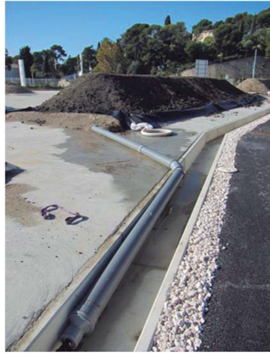
Fig 3. Pilot landform and its percolation collecting system
